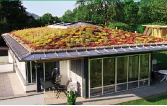
Extensive greening on flat and pitched roofs
