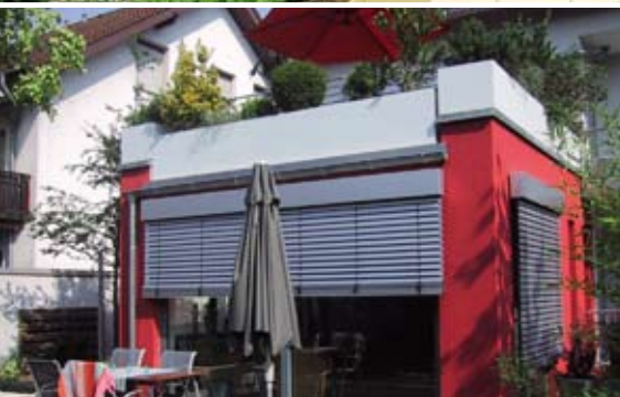
Plant containers as boundaries with railings
