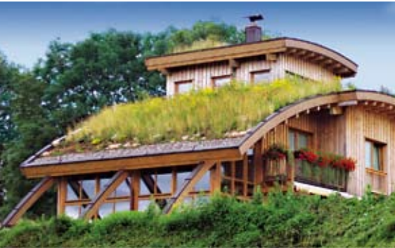
Extensive greening on steep roofs
